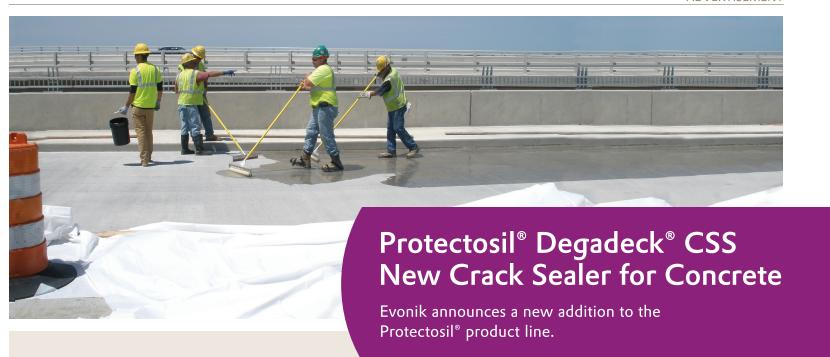
Protectosil® Degadeck® CSS is a two component, low viscosity methylmethacrylate (MMA) resin for use on horizontal concrete surfaces. Protectosil® Degadeck® CSS is formulated to have excellent penetration into the crack while maintaining high compressive and flexural strengths. In addition, the product cures quickly to minimize the time in which the traffic lanes or parking decks need to be shut down for repairs.
