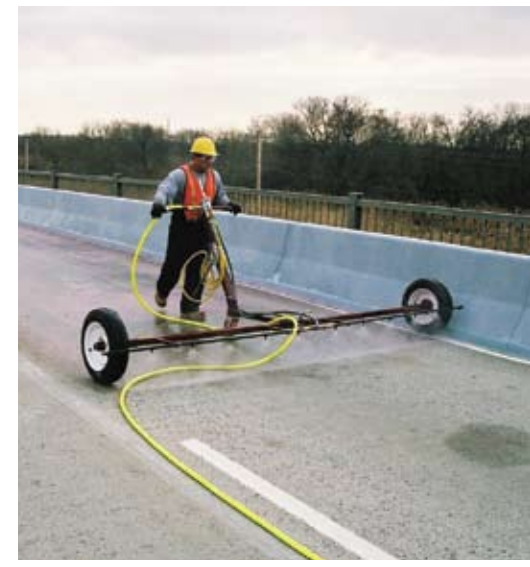
* Photos of spraybar application on the bridge span of the Commodore Barry Bridge.
